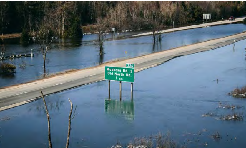
◀ Highway 11 inundated by flood waters during the “Cottage Country Flood” in 2013
